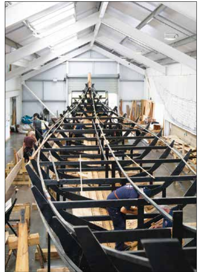
WOOD AND COULD: Volunteers work on the replica of the Sutton Hoo longship in Woodbridge, Suffolk. Three apprentice joiners are undertaking a two-week-long placement with the Sutton Hoo Ship's Company, which is leading work on the 88ft-long full-size replica
