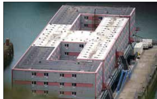
HEALTH HAZARD: The Bibby Stockholm in Portland Port, Dorset
